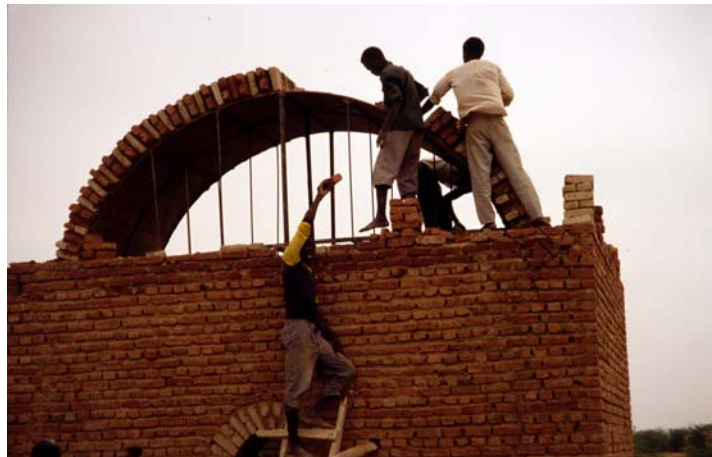
Figure 5: Bricks being used in the construction. Photo: Practical Action / Mohammed Majzoub
